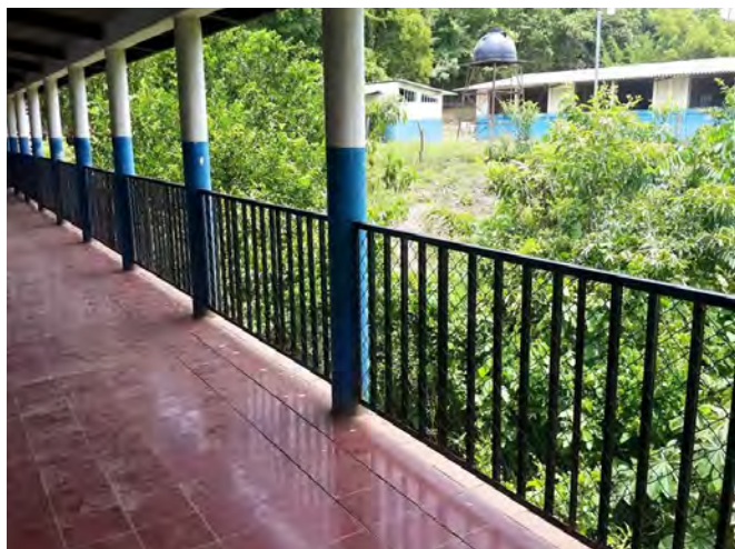
Our donations paid for this new railing by the kindergarten classroom
